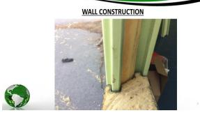
**SMARTSTEEL IS 12" OF FOAM INSULATION SANDWICHED BETWEEN TWO SHEETS OF 22 GAGE GALVALUME STEEL TO ACHIEVE A PHENOMINAL R-RATING OF 49. 25% ELECTRICAL ENERGY REQUIREMENT COMPARED TO CONVENTIONAL** CONSTRUCTION.
